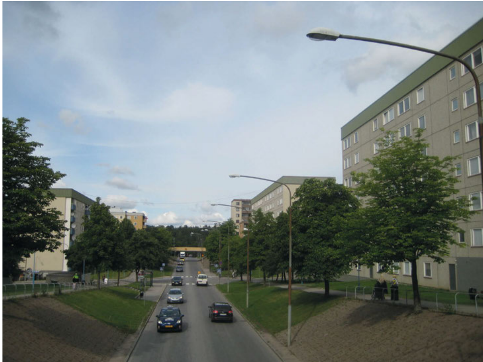
Igor Dergalin was inspired by Venice's bridges and canals whilst planning Tensta-Rinkeby's traffic separation with bridges for pedestrians and tunnels for motorists.
