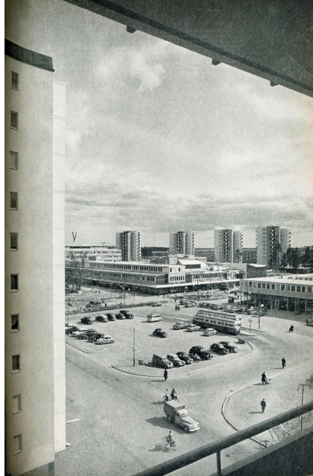
View over Vällingby Centrum in 1956 with Hjalmar Klemming's the tall point blocks surrounding Vällingbyplan Square, Reinius and Backström's low shopping architecture with the restaurant Vällingehus sticking up. Car-ownership quickly accelerated after the picture was taken, so the centre had to expand. Markelius, Sven: "Stockholms Struktur. Synpunkter på ett storstadsproblem", in Byggmästaren , 1956, A3.
