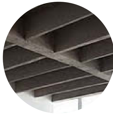
concrete reinforced ceiling
