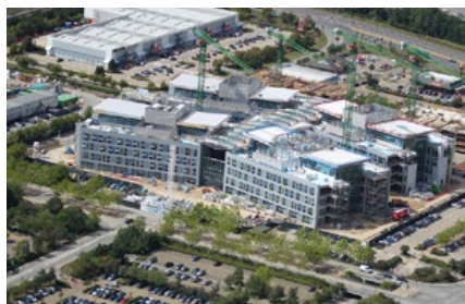
The Quadrant under construction.
