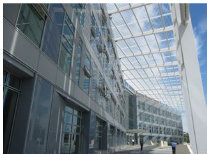
Sunshading the external structure.
