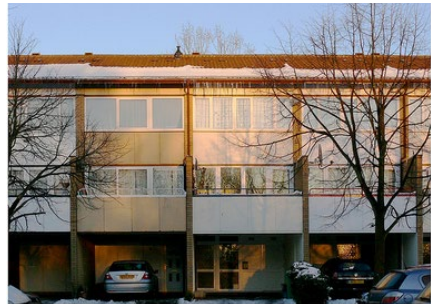
Original and current situation of the housing
