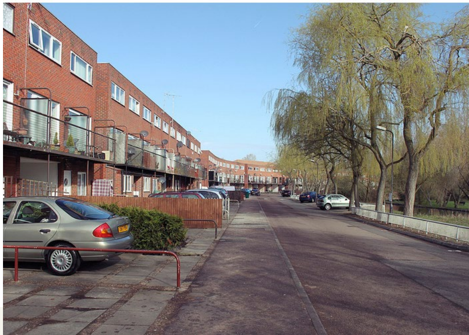
TYPICAL Milton Keynes Development Corporation
