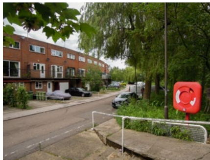
Safety equipment at the canal
